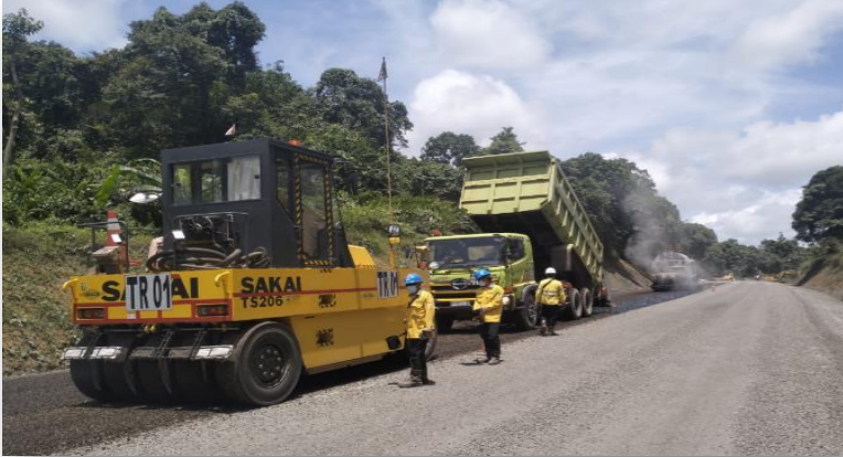
Hauling Road Upgrade
